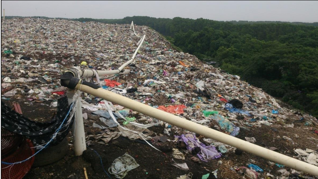
Figure 23: Existing landfill gas recovery system on cell 1. This system is a vertical system.
